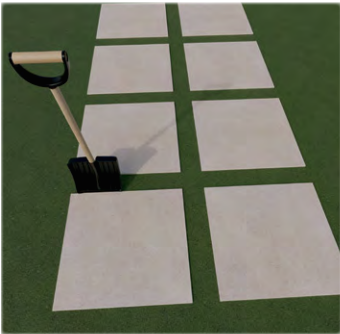
1- Dry installation on grass Installation on the ground without leveling layer and regularization of cement mortar. Ideal for garden areas.
