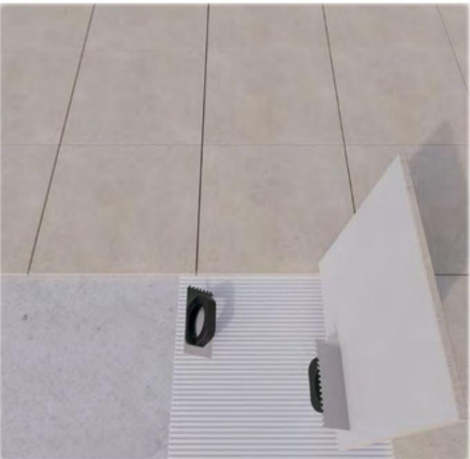
4- Thin-bed installation with cementitious adhesive Installation in terraces requires qualified personnel. It is only recommended to employ professionals with proven experience in this type of work.
