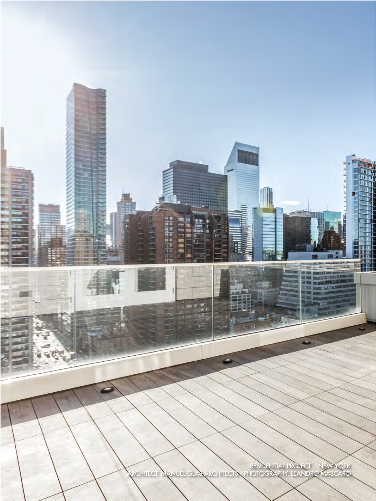
Raised Access Flooring outdoor
